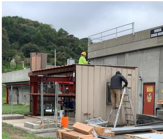
SBS Spill Containment Vault Under Construction
