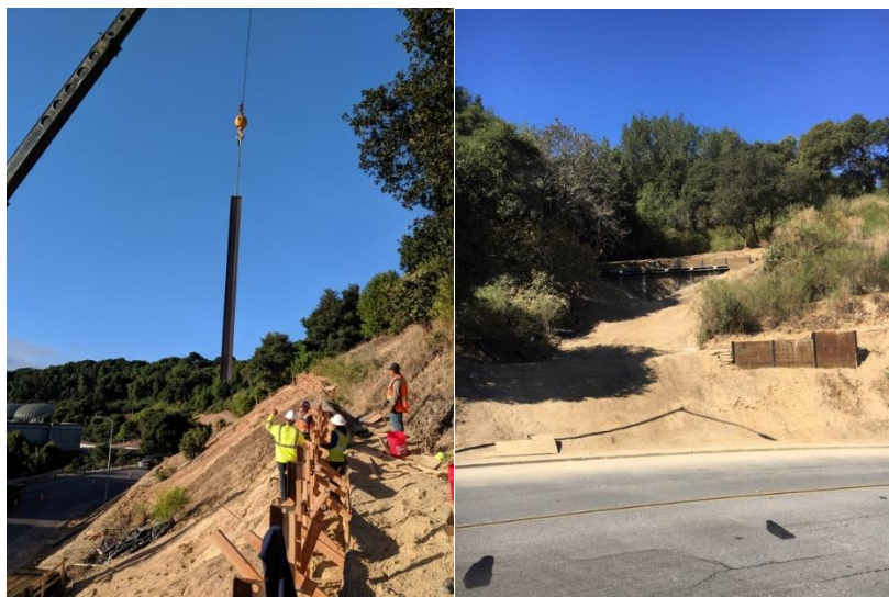
Retaining wall construction
