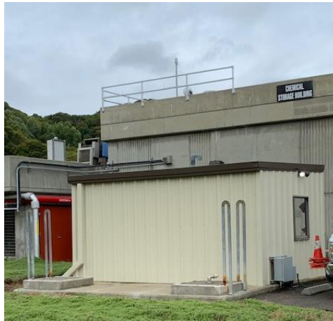
SBS Spill Containment Vault after Refurbishment
