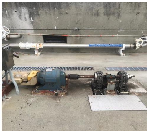
Removal of Original Drive Assembly
